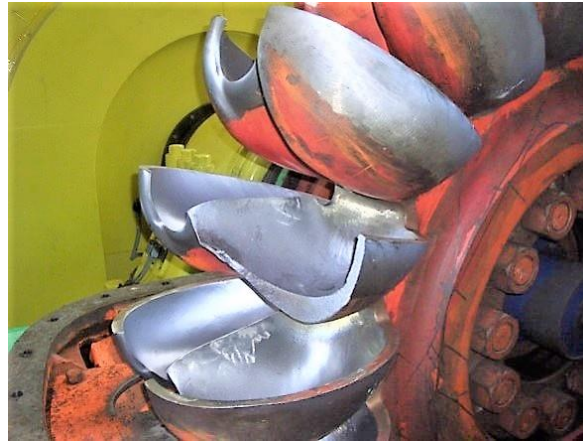
Figure 8 Damage in a bucket
