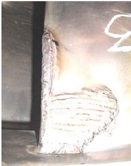
Fig. 12. Cavitation damage in a turbine blade.
