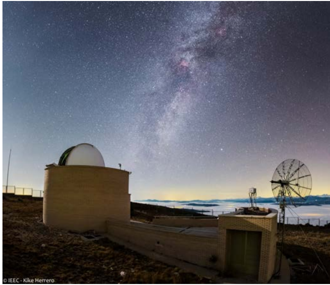
Figure 9.2: S-band antenna used to download FMPL-2 scientific data, located at the UPC/IEEC Montsec Ground Station.
