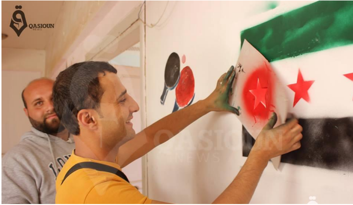
80- Al Atareb Local Council paint the revolution flag on public building - Source : Qasioun Net
