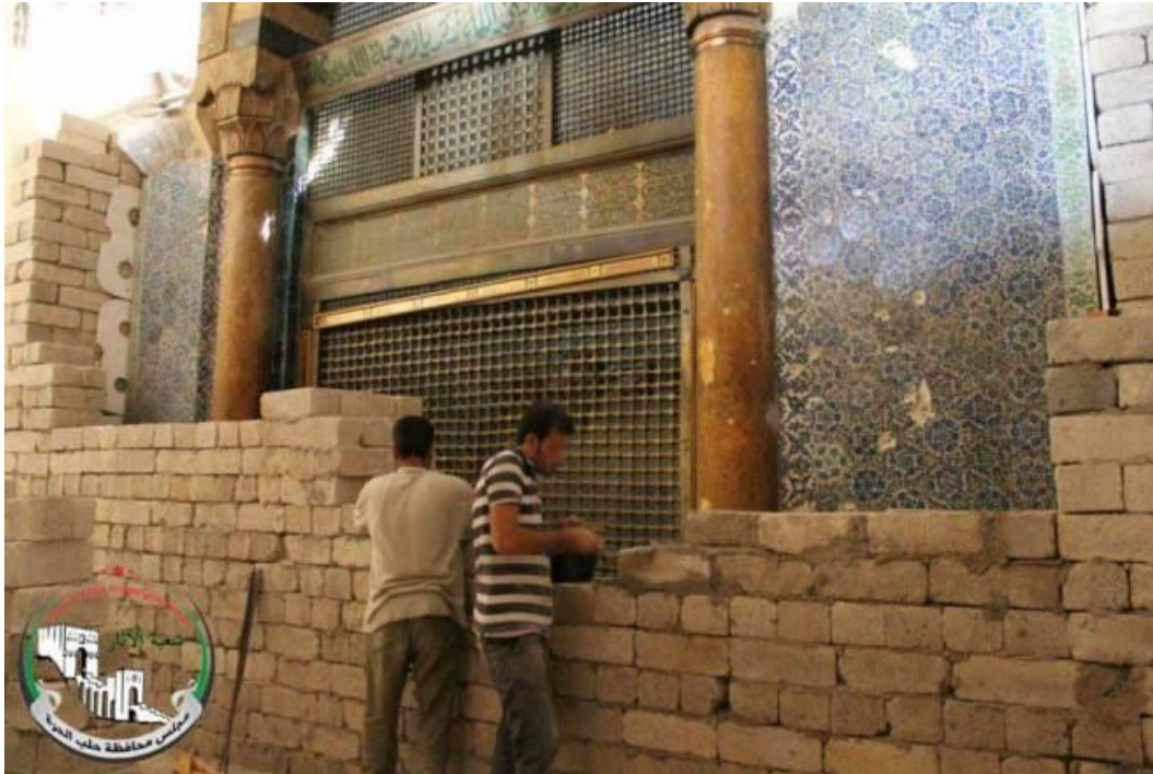
61 – Works of protection of Meqams at the Great Umayyad mosque by Aleppo Provincial Council - Source: the Council's Facebook page
