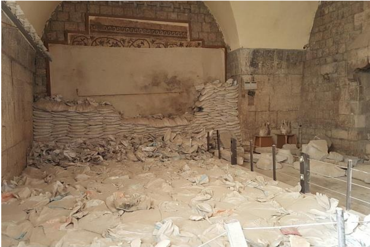
65- Several truckloads of sand bags were delivered 2014-15 to protect the Ma'arra Museum mosaics from damage caused by further attacks – Source: the Penn Cultural Heritage Center
