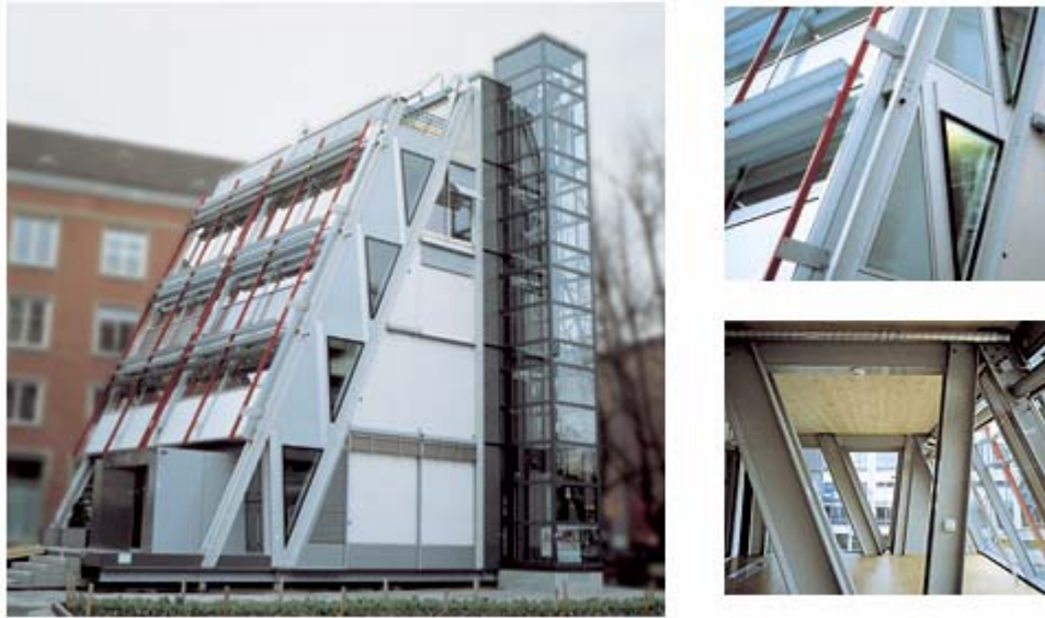
Figura 2.14. The Eyecatcher Building
