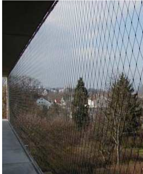
Figura 87. FacadeScape system. X-Tend Stainless Steel Flexible Mesh Fabric. Carl Stahl Décorcable [6], [7]
