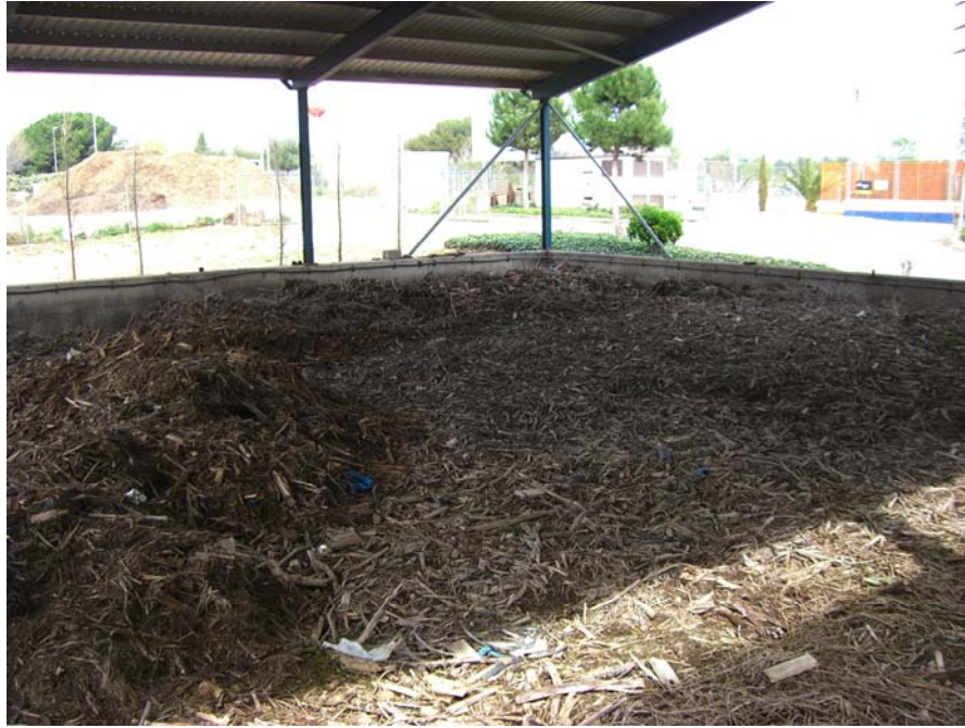
Figure 7.2. Detail of the Biofilter 2 (first day of analysis) at the anaerobic digestion and composting plant.
