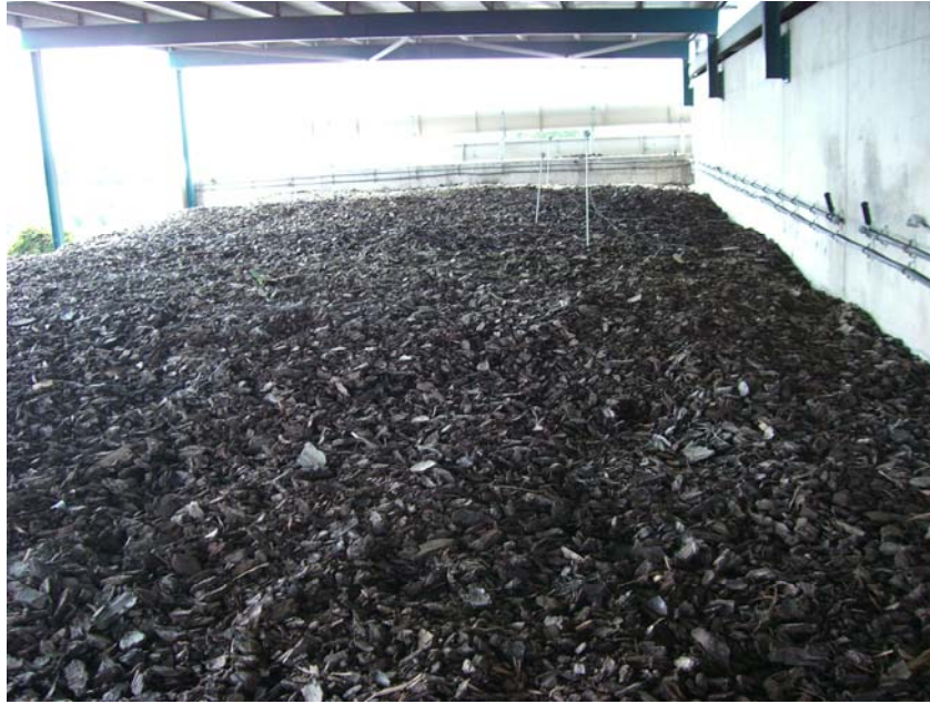
Figure 7.4. Detail of the Biofilter 1 (first day of analysis) at the anaerobic digestion plus composting plant.
