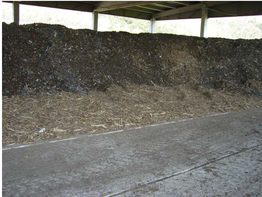
Figure 6.3. Maturation area at tunnel composting plant. Detail of the absorbent layer and perforated pavement.
