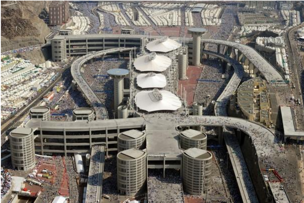
The New Jamarat Bridge.
