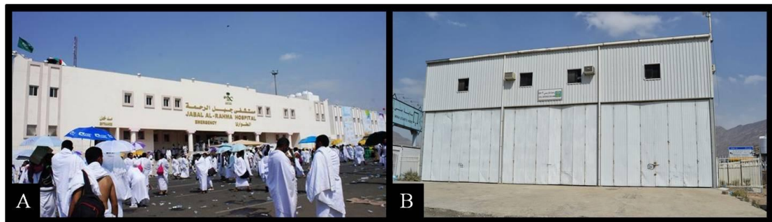
A) One of the Hospitals Buildings in Arafat, B) Fire Station Steel Structure.
