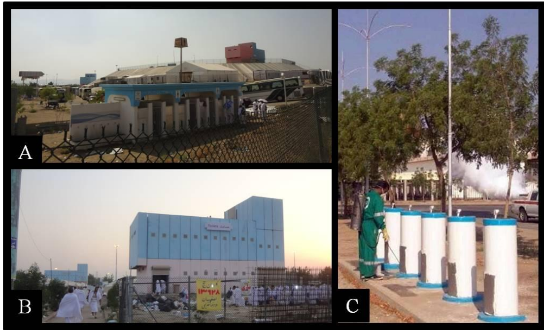
A) the Old Model of Toilet Complexes, B) the New Model of Toilets Complexes in Arafat and C) The Public Drinking Water Fountain.
