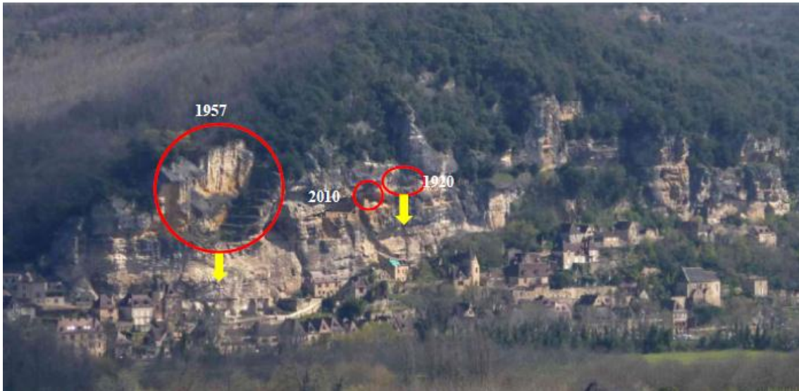
Figure 8.200: Location of the resent landslides
