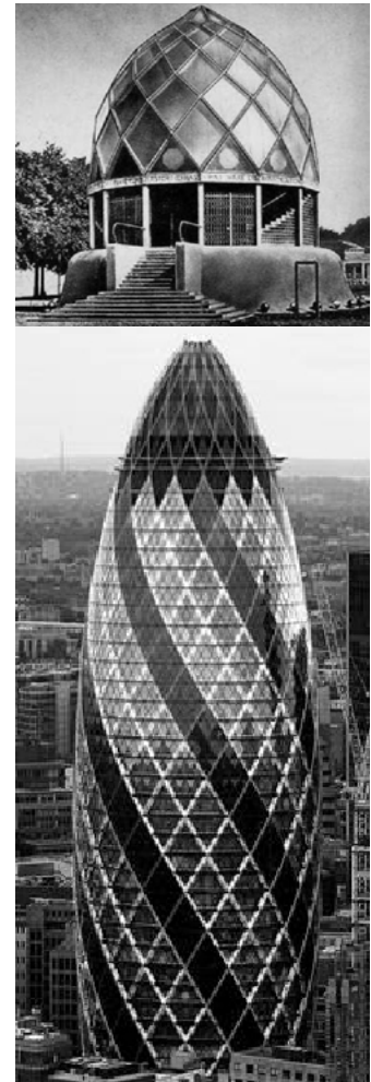
Fig. 2-22: (Superior) Taut Glass Pavilion, Cologne, Germany, Bruno Taut, 1914 . (Inferior) Swiss Re Headquarters, Londres, Foster & Partners, 1997-2004.
