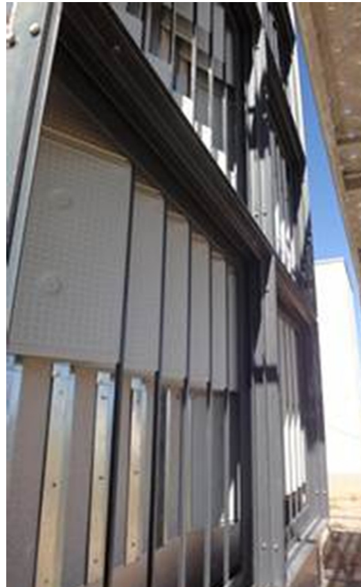
Fig. 4. PCM distribution inside the air chamber.
