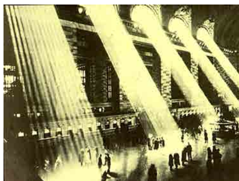
Fig. 42. Central Station. Nueva York, 1871.
