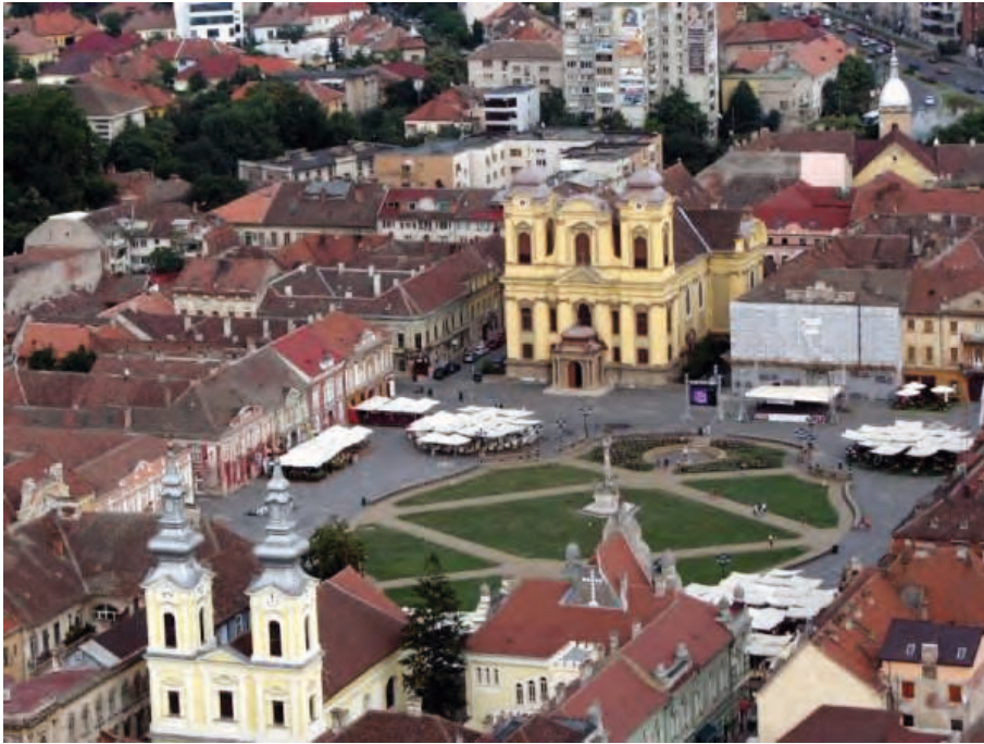
Figure 3.36: Urban experiment – Overview of the Unirii Square. Aerial view of the Unirii Square.
